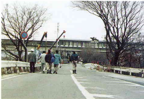
(a) 堤防天端の波打ち
