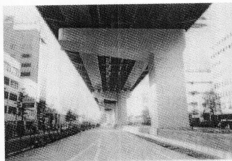
Fig.1 Inverted L-shaped steel bridge pier (Nagoya Expressway)
