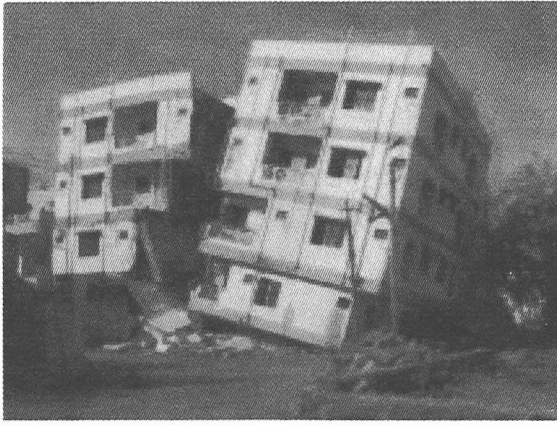
Figure 9: Failure of RC buildings due to soft-floor effect in Bhuj
