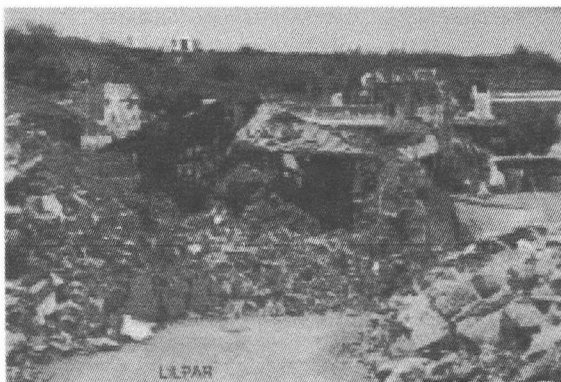
Figure 5: Collapsed masonry buildings in Lilpar
