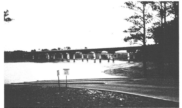
写真－9 View of I-75 southbound over Lake Allatoona
