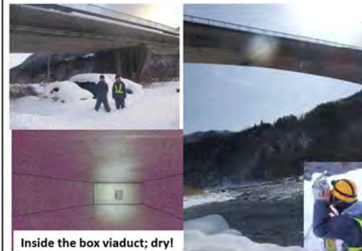
Inside the box viaduct; dry!
