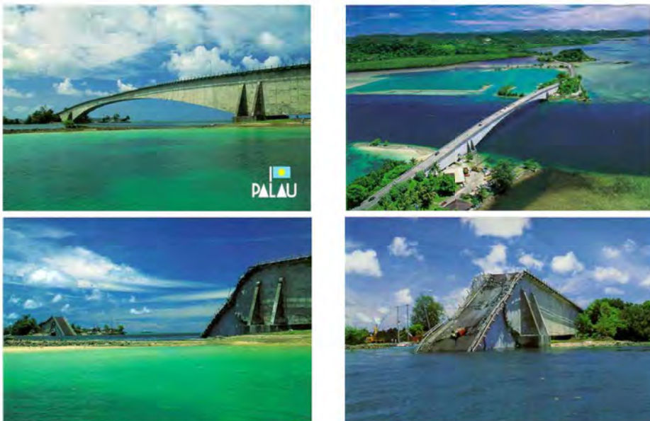
Given by Prof. Bazant for academic use (Northwestern University, Home-page) Palau: Koror-Babeldaob bridge. Sudden Collapse at 20 year after construction
