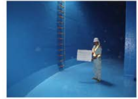
Water Proof in the Elevated Tank
