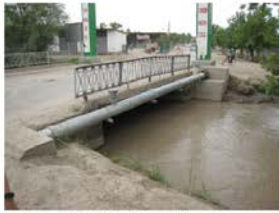
Transmission Pipe (Pipe Culvert at River Crossing)
