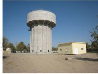
Elevated Tank for Pyanj Town and the Adjacent 3 Villages (1,800m 3 )
